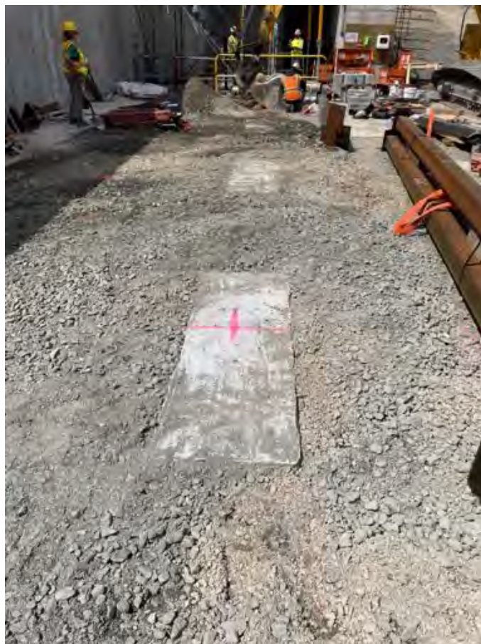
Deadmen in place.
