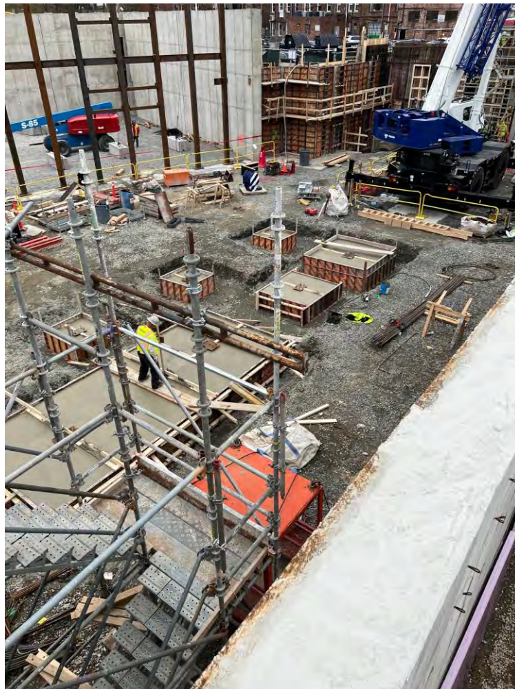
Interior footings, Area A.
