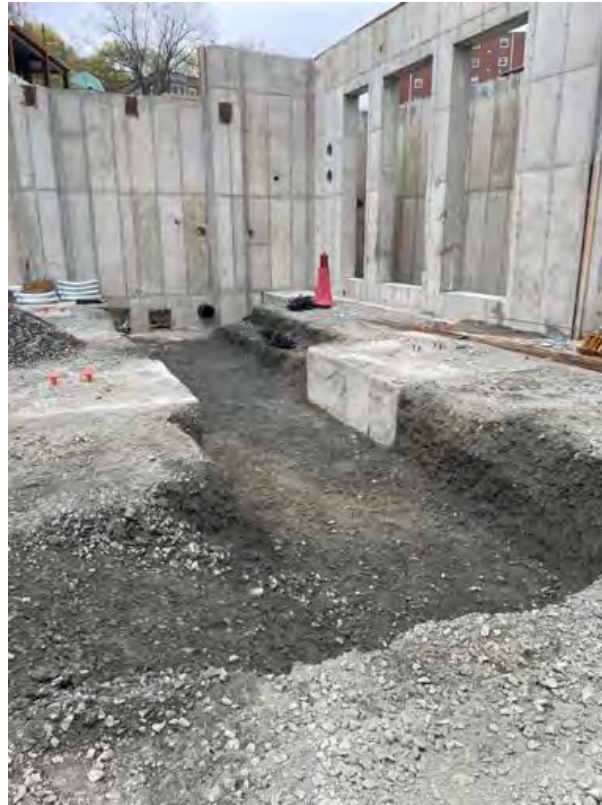
Excavation for electrical ductbank.
