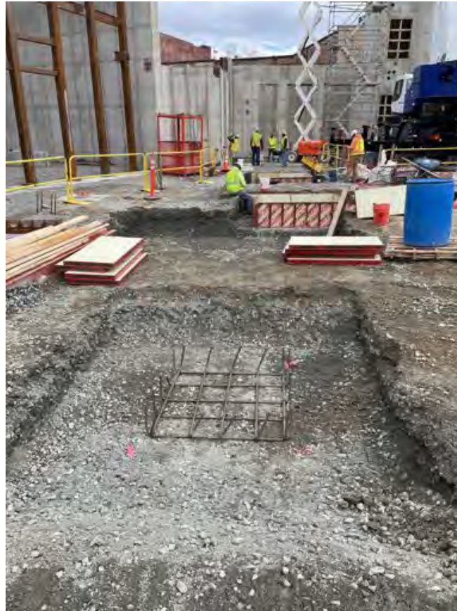
Excavation for interior footings.
