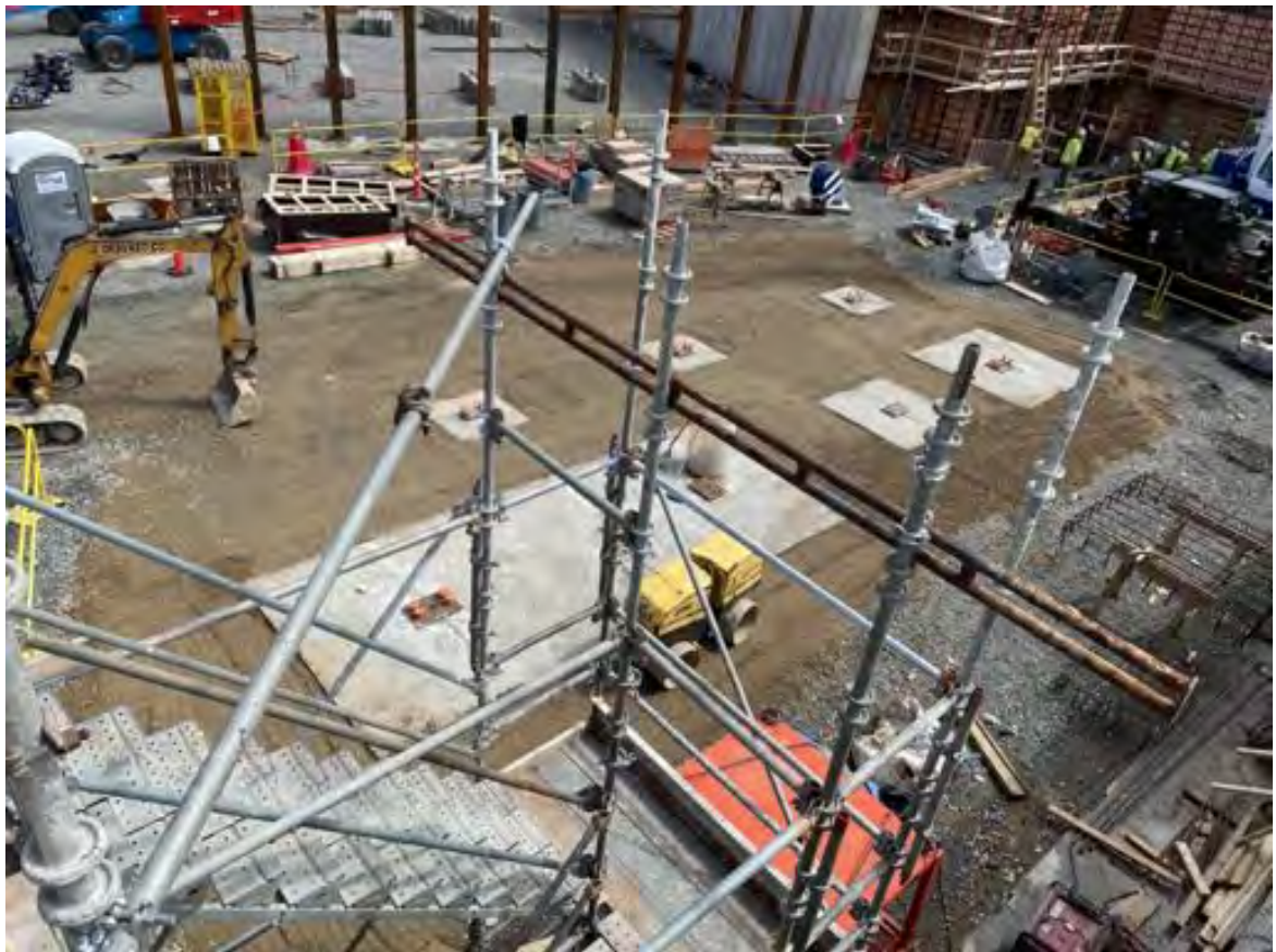
Backfill and compact at interior footings.
