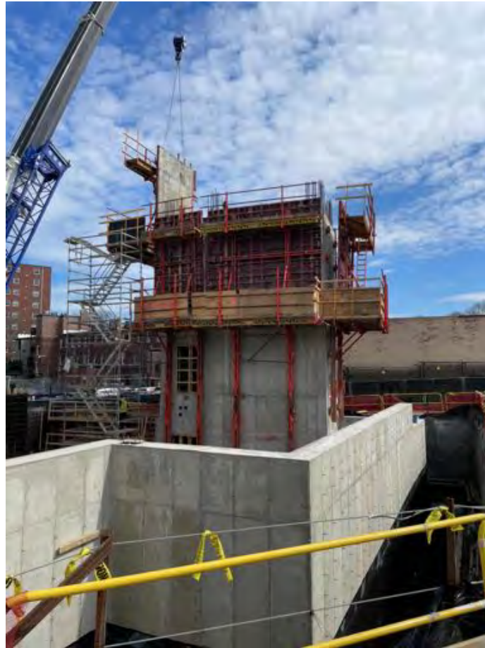
Releasing and raising forms, Core A level 2 to 3.
