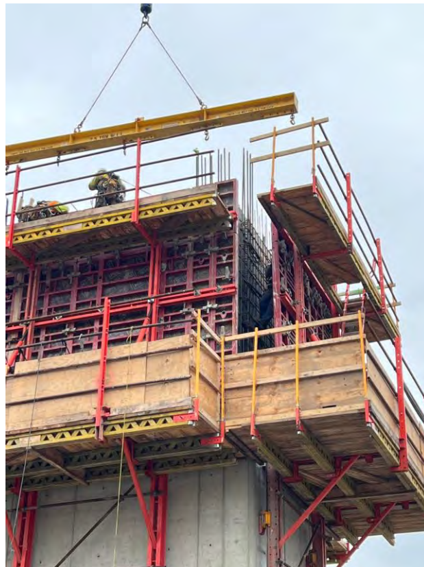
Installation of Rebar at Core A level 3
