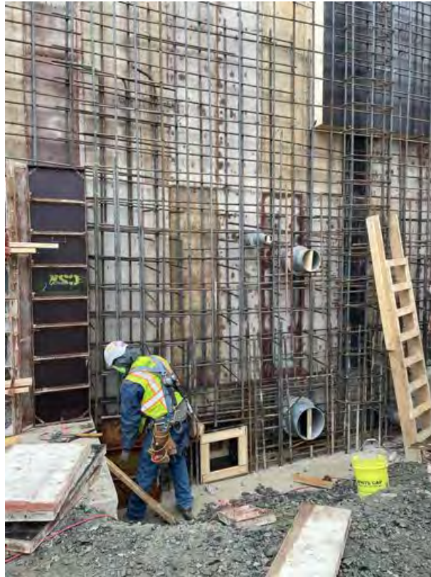
Sleeves and rebar at line AR wall.
