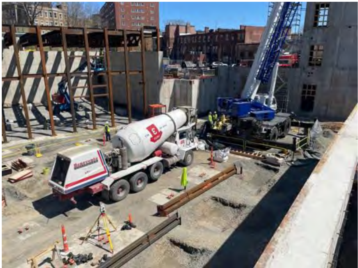
Interior footings; forms, rebar, concrete.
