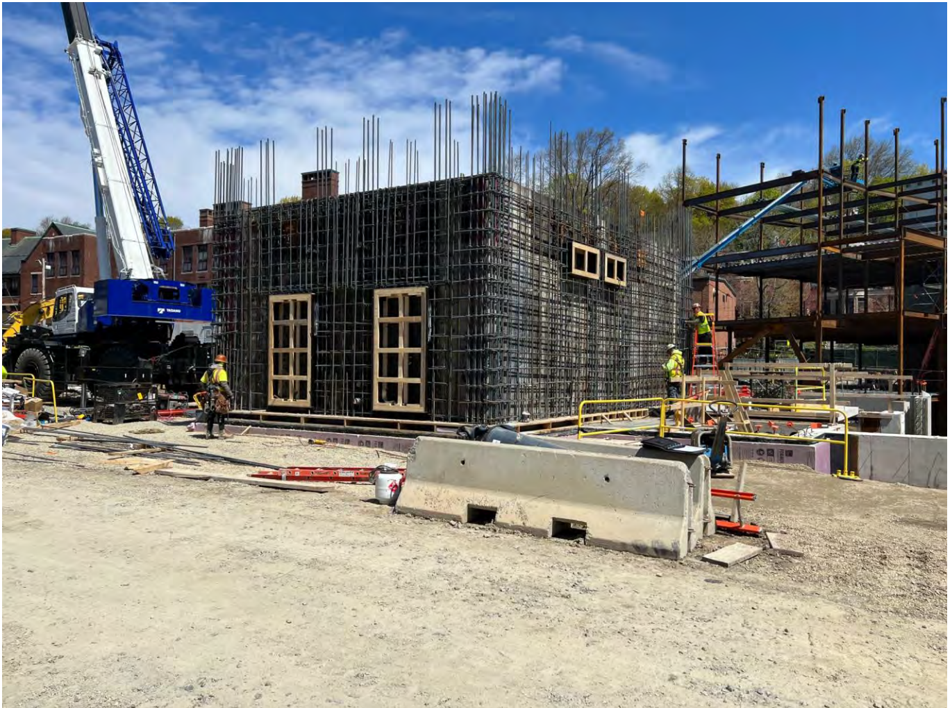
Core AB forms, rebar and embeds.
