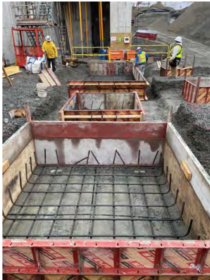
Interior footings, Area A.
