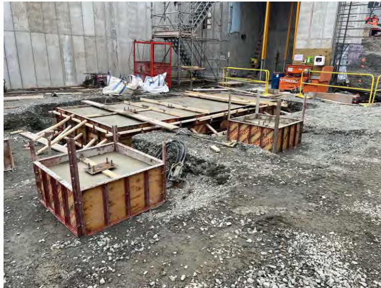
Interior footings, Area A.
