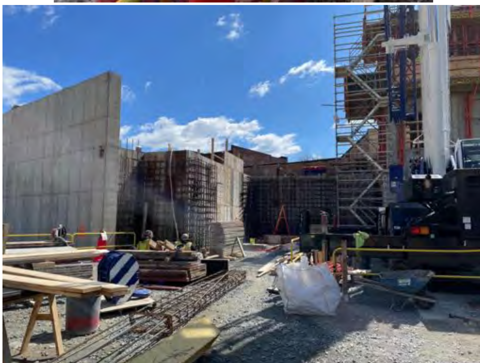
Forms and rebar along line AR.
