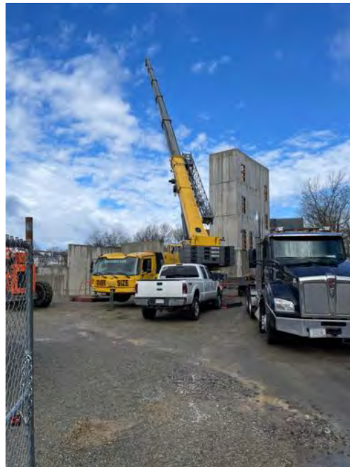
Set and prep steel crane
