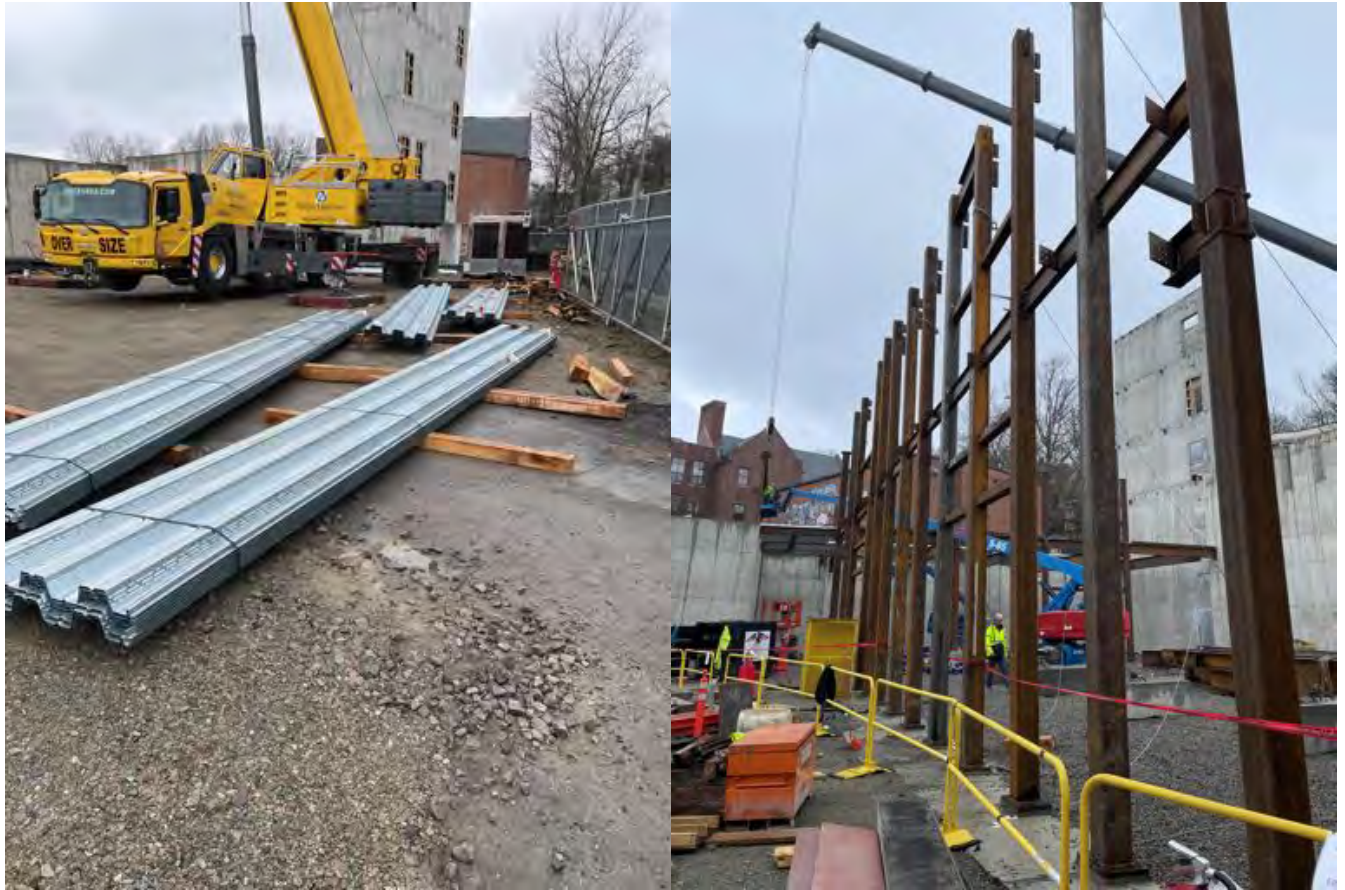
Steel installation ongoing, Sequence 102.
