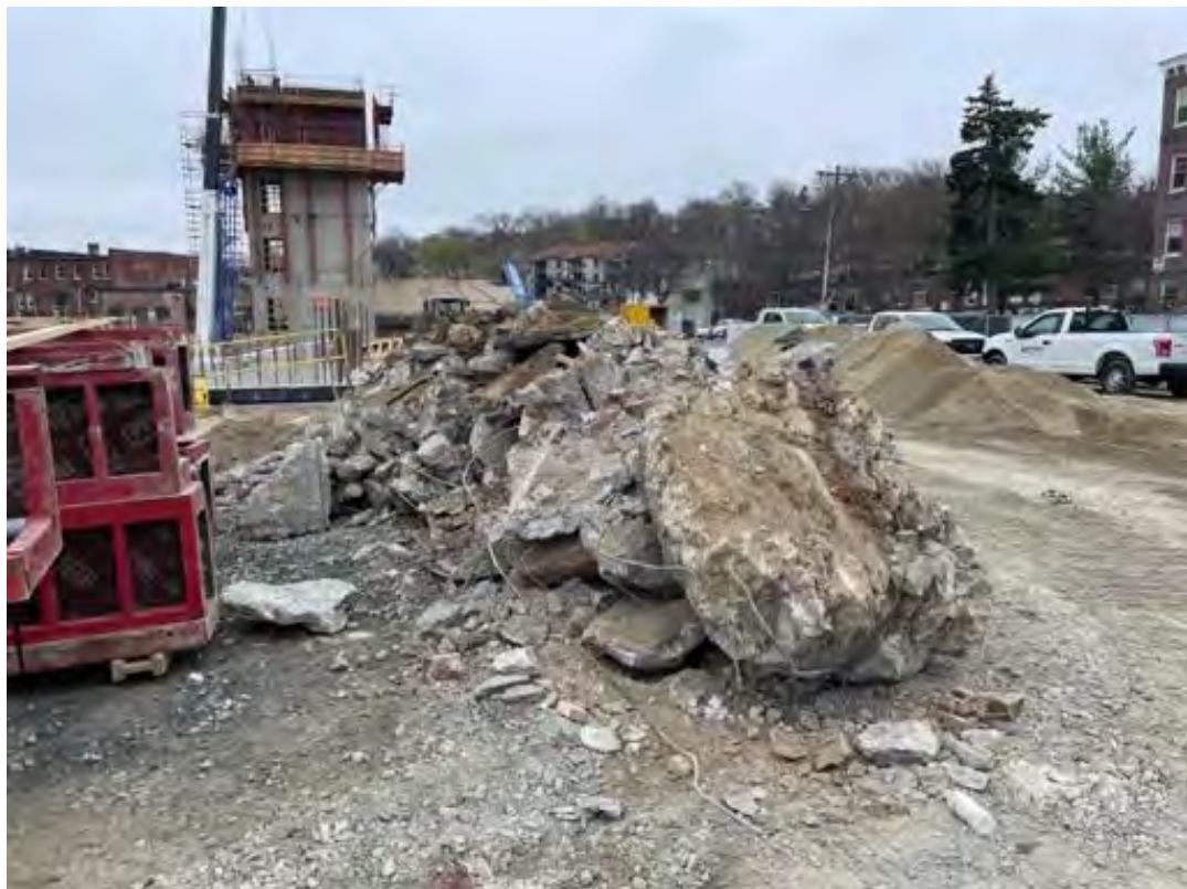
Rubble from partially demolished SOE.
