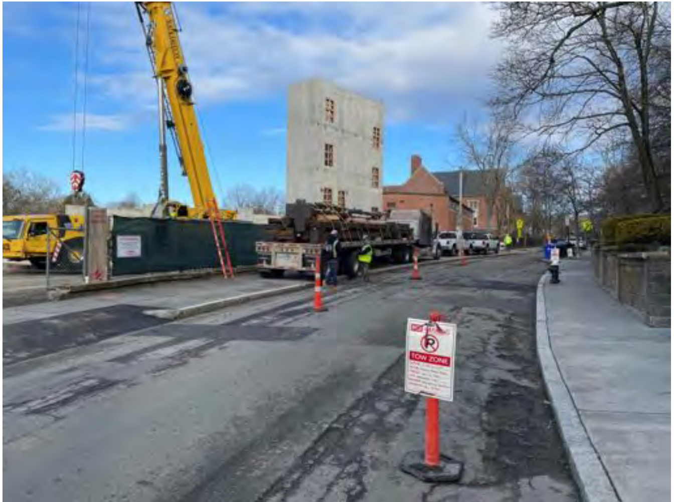
Sidewalk on Westbourne Terrace closed for steel deliveries. Police details in place.
