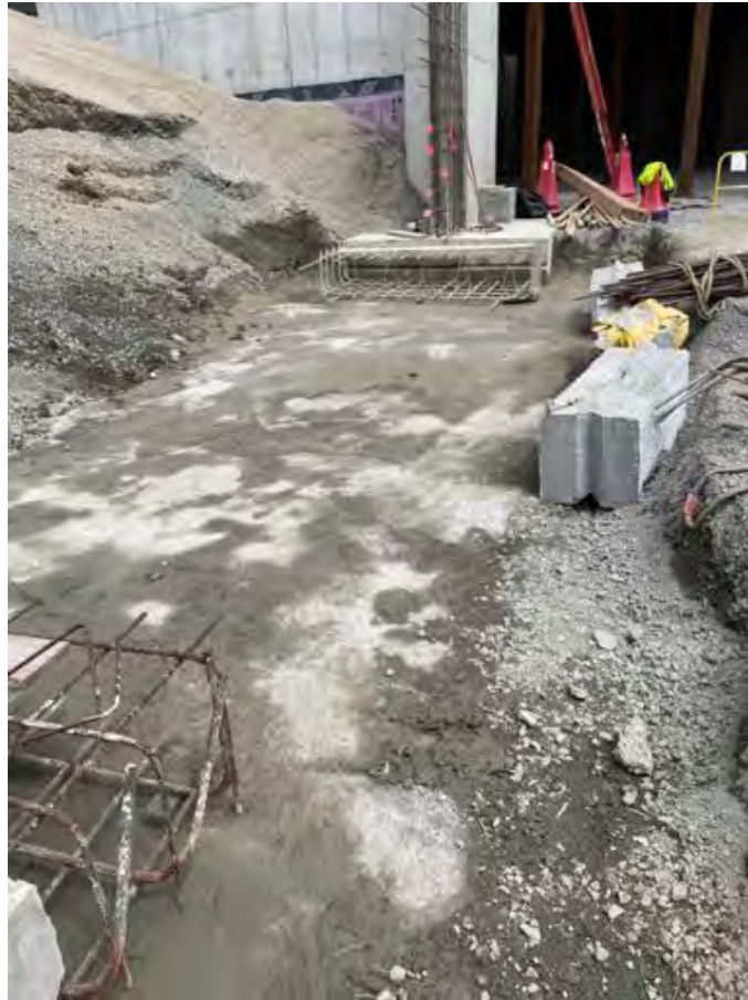
Removing the ramp and excavating for footings.
