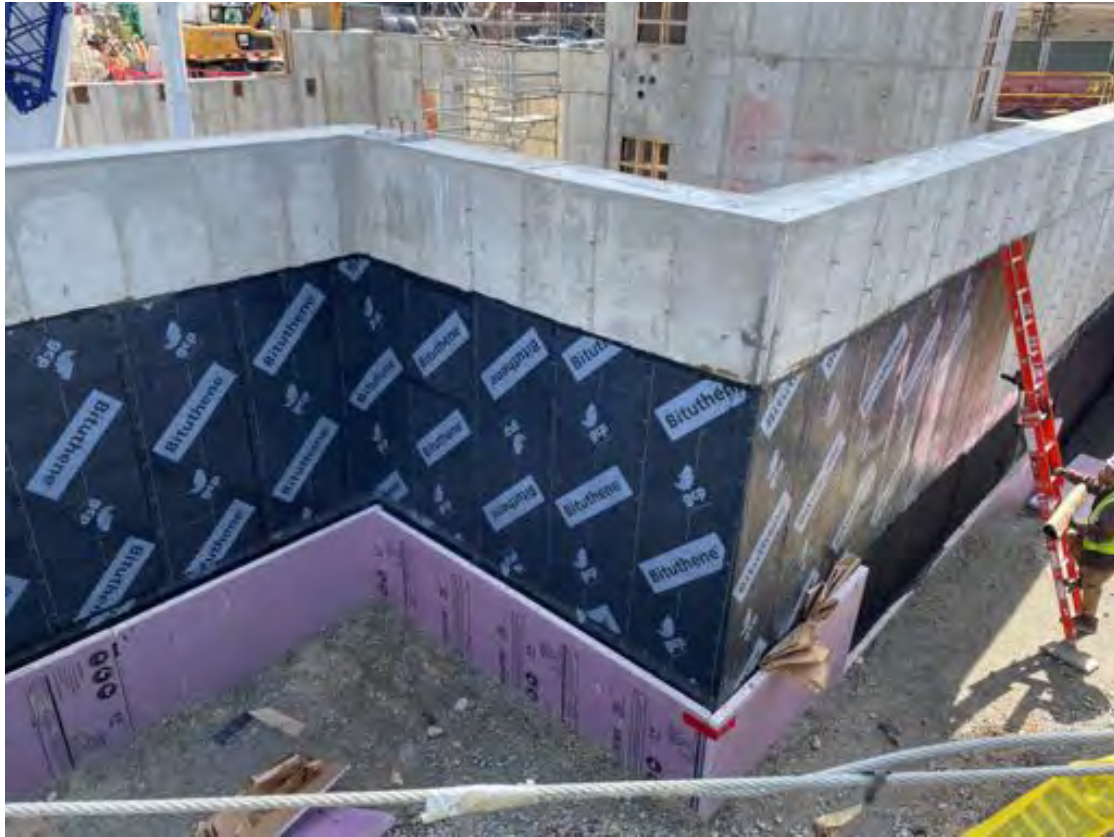
Waterproofing along line AG.
