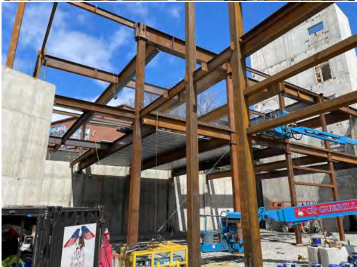
Spreading out metal deck.
