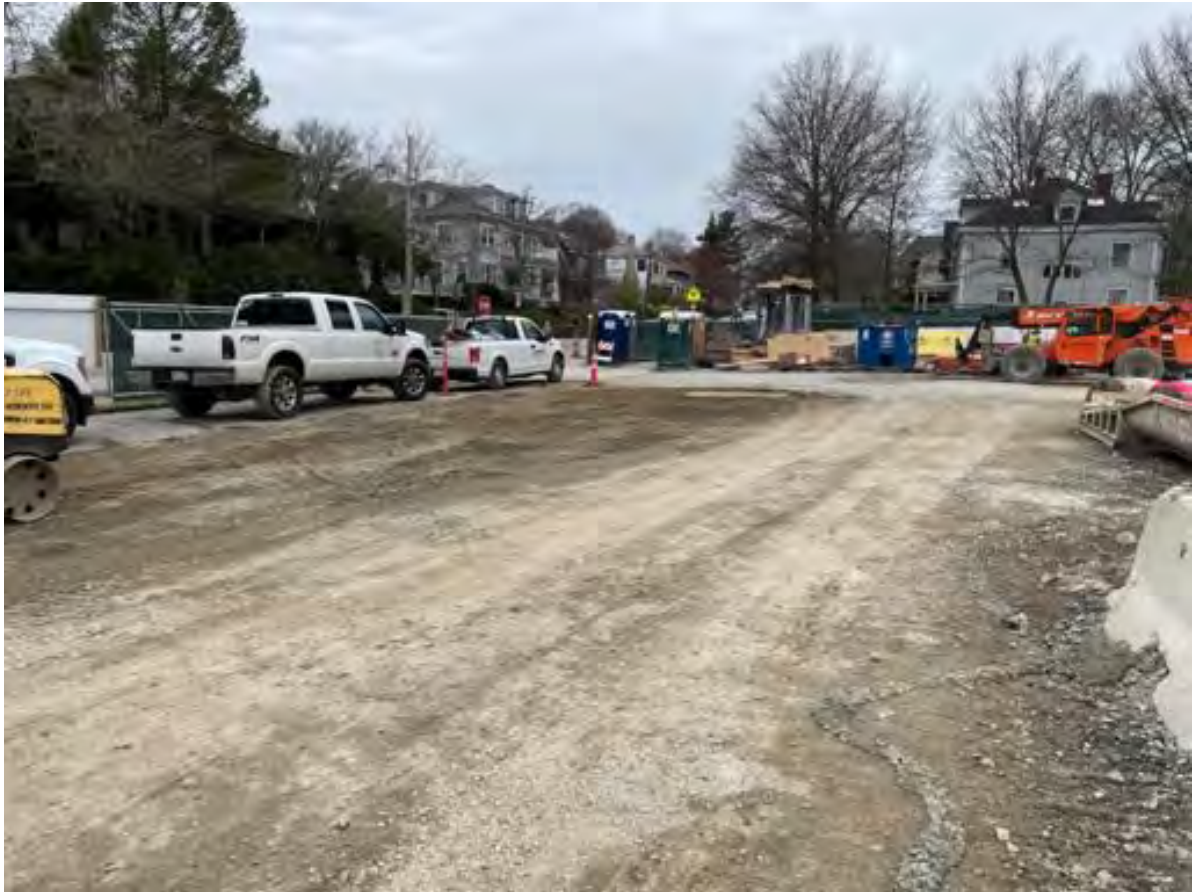
Signal box removed at Washington St.
