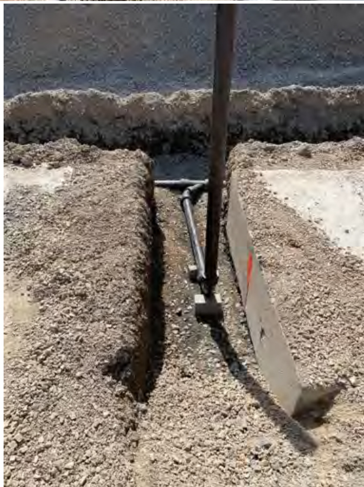
Underground plumbing, Area A.
