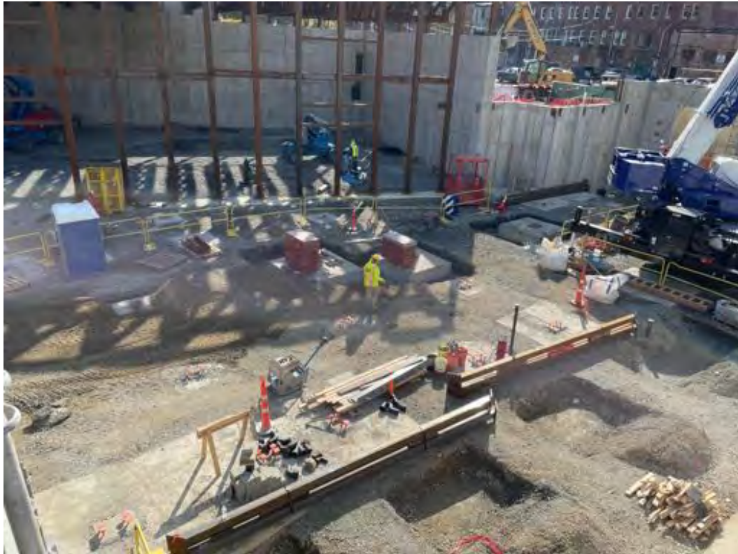
Interior footings backfilled.
