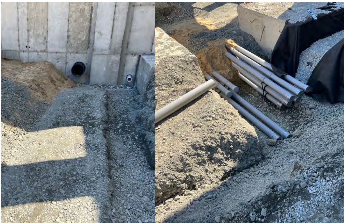
Electrical ductbank being backfilled.
