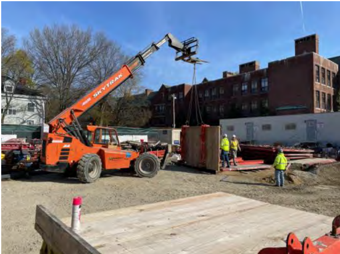
Building forms for Core AB.
