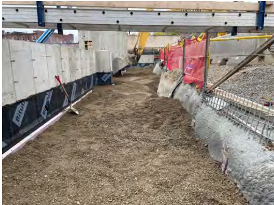
Waterproof, backfill and compact along line AG.
