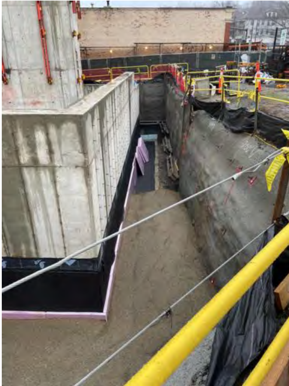
Backfill at line AG.
