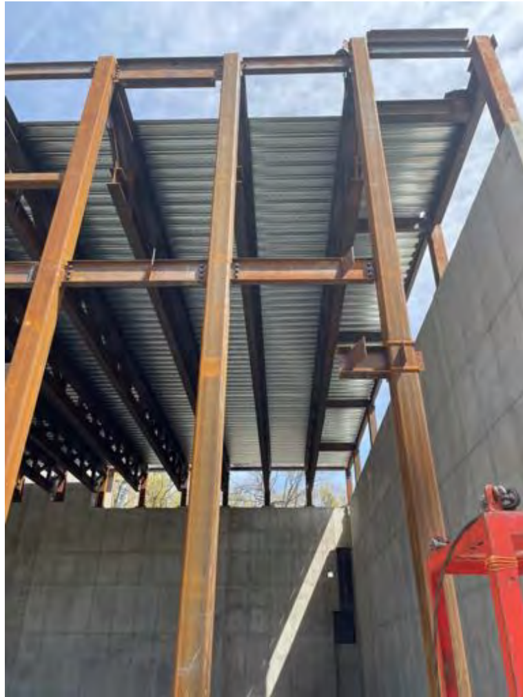
Steel decking above gym.
