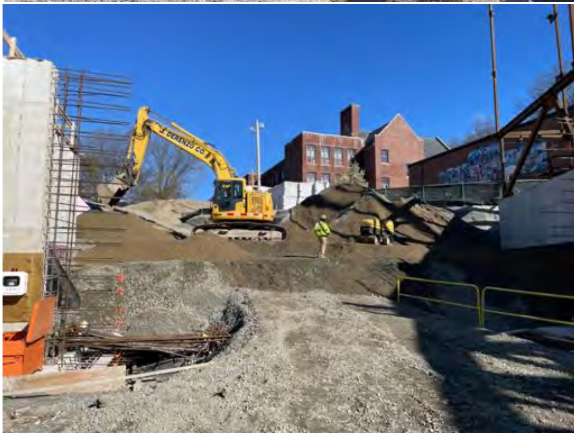
Backfill and compact ramp area.
