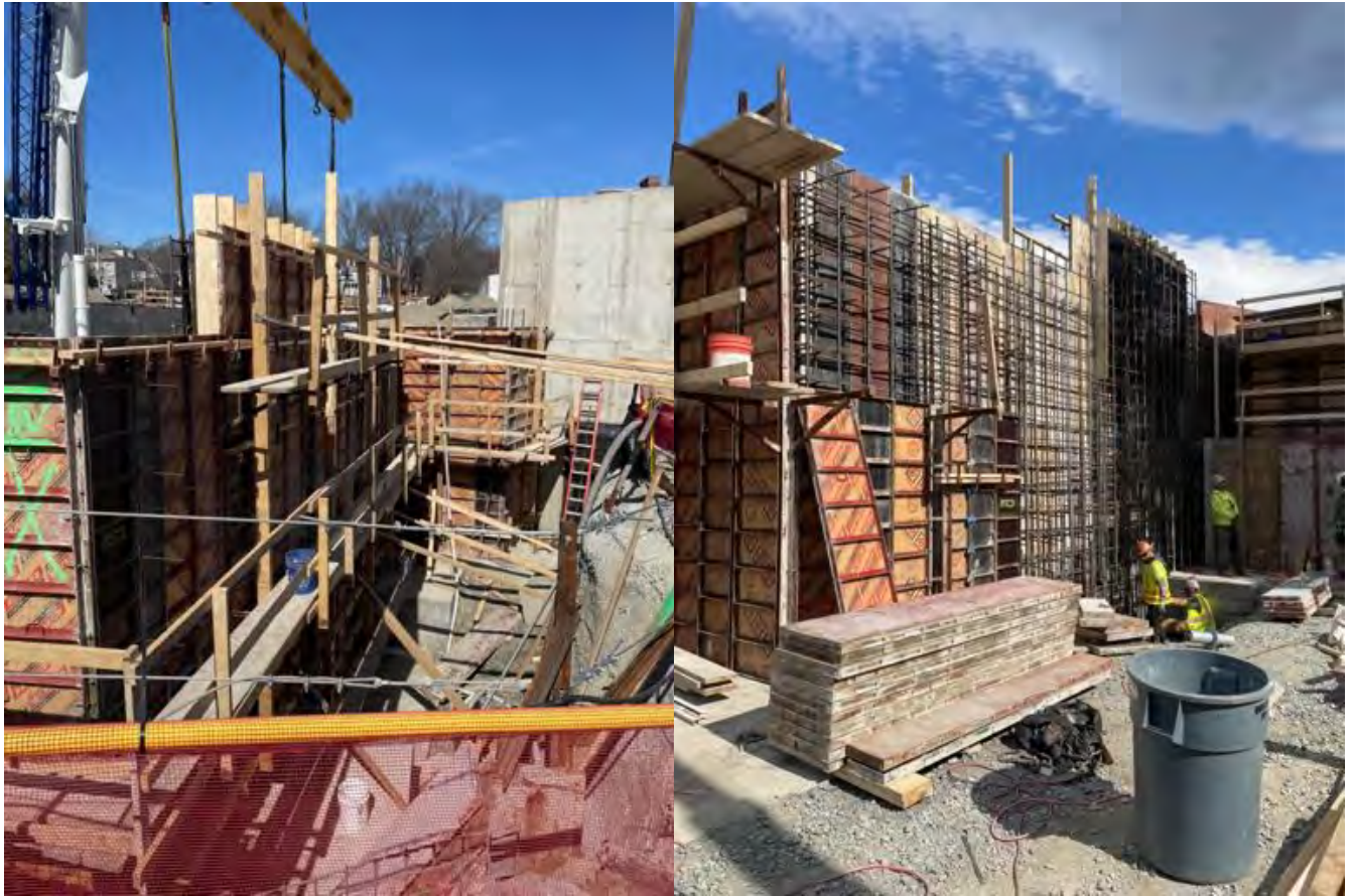
Forms and rebar, line AR.
