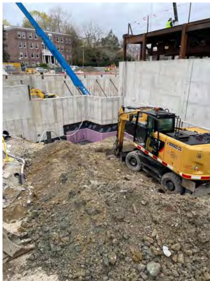
Excavation and lean concrete on East side.
