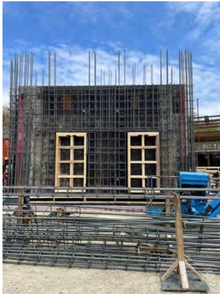
Core AB forms, rebar and embeds.
