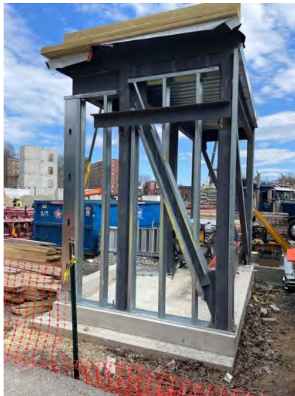
Metal framing at mock-up
