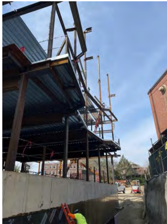
Steel, West side.
