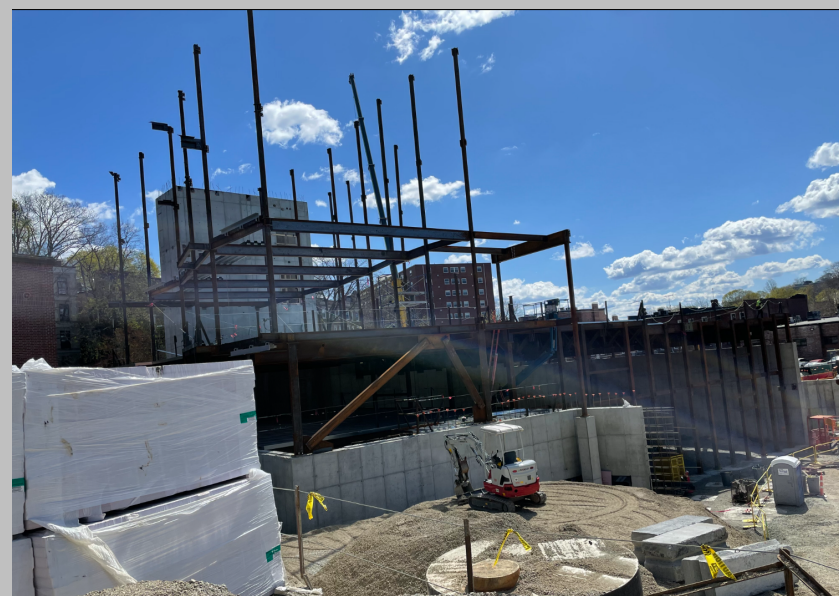
Building C- Steel Erection
