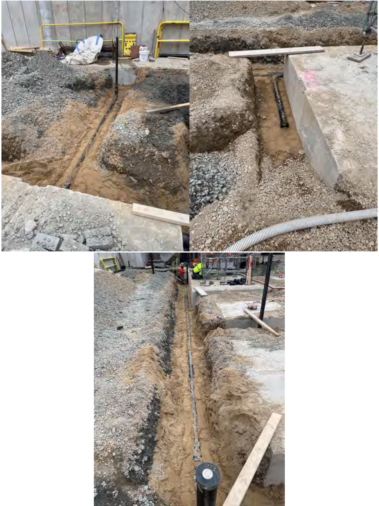
Underground plumbing, Area A. Plumbing inspection passed.
