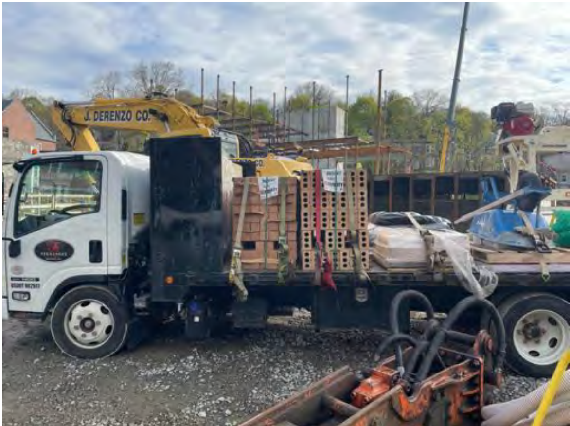
Deliveries – pipe and masonry.
