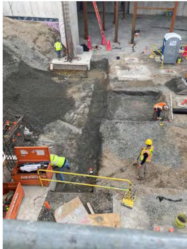
Removing the ramp and excavating for footings.
