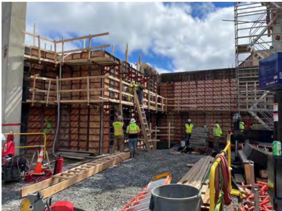
Forms at line AR completed.
