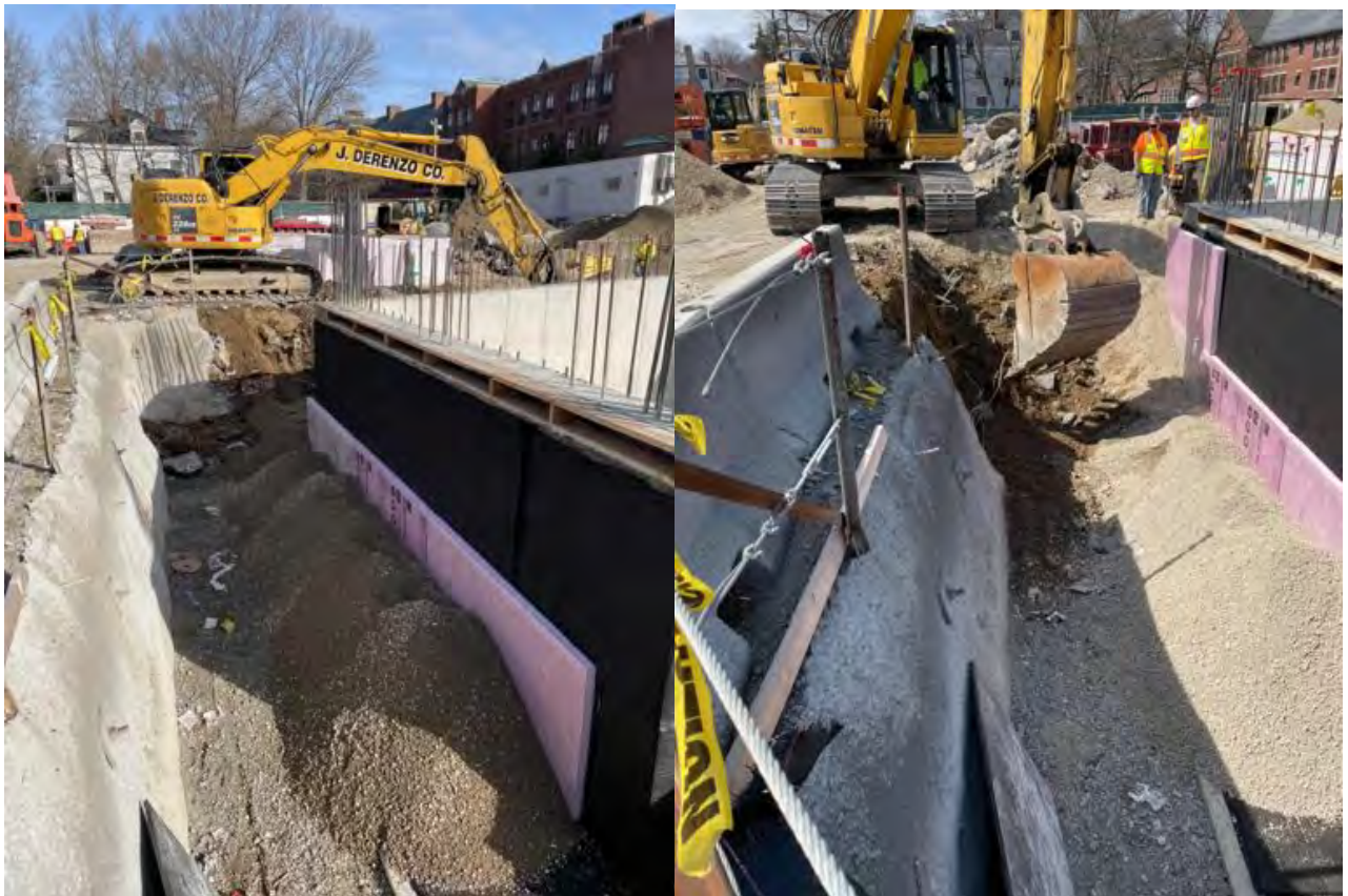
Backfill and compaction, Core AB
