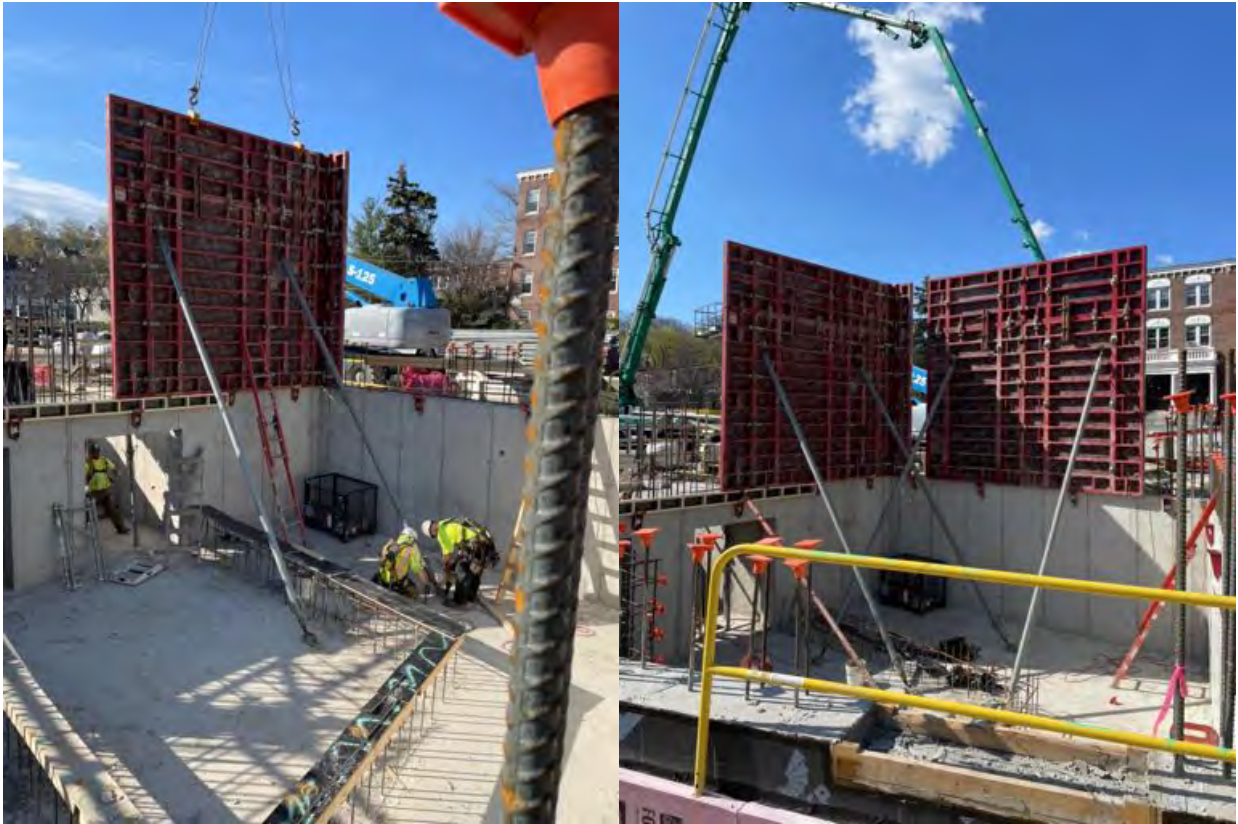
Setting forms for Core AB.
