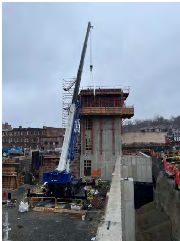
Core A forms at level 3.
