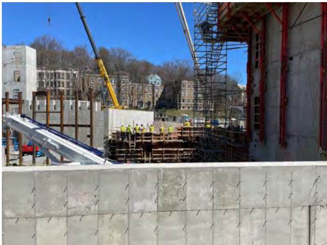
Concrete pour, line AR.
