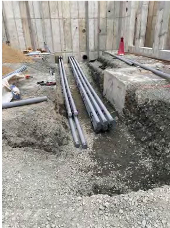
Electrical ductbank.
