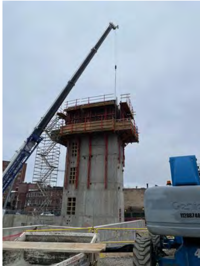
Core A forms raised, rebar installation ongoing.
