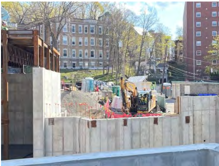
Work on East side.
