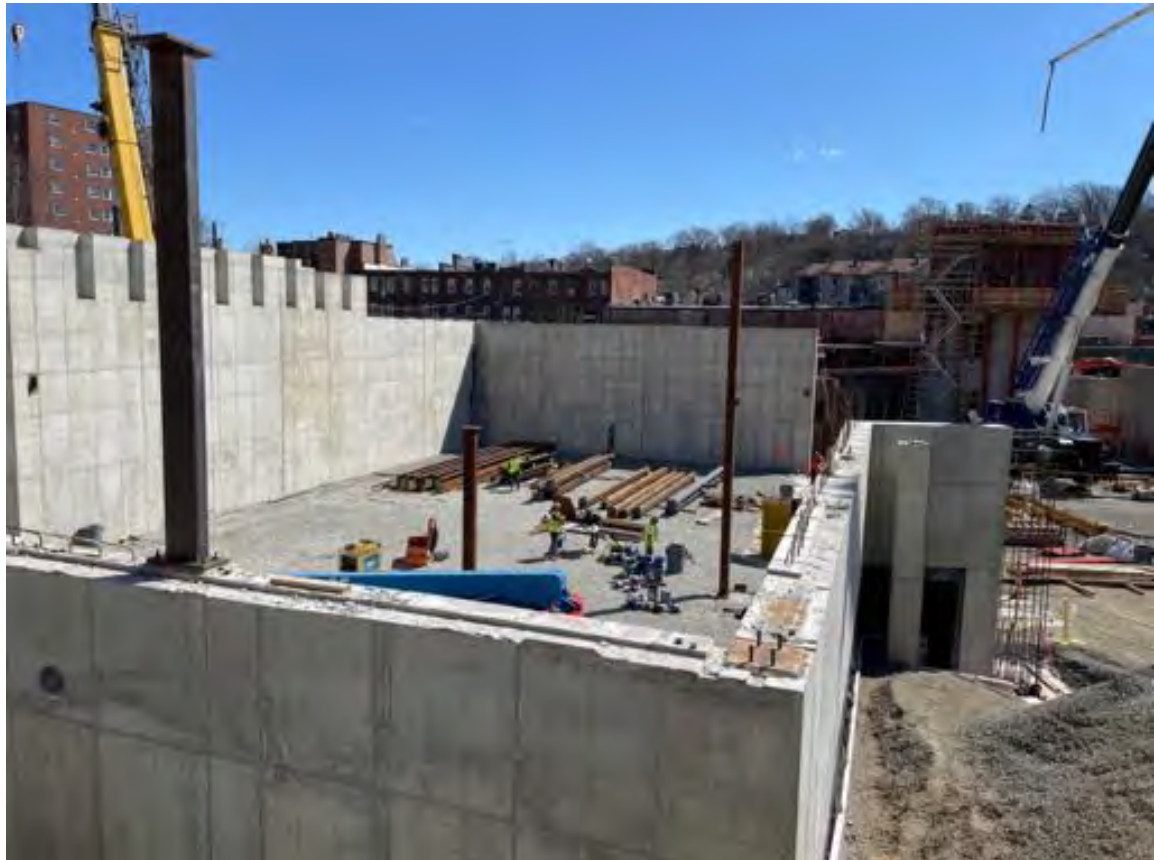
Shaking out and setting steel.
