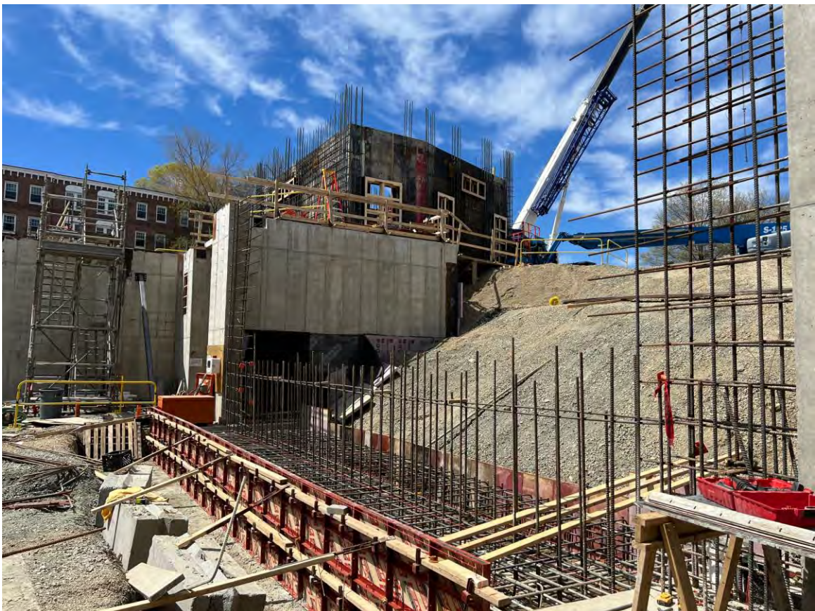
Forms and rebar being installed along line A1
