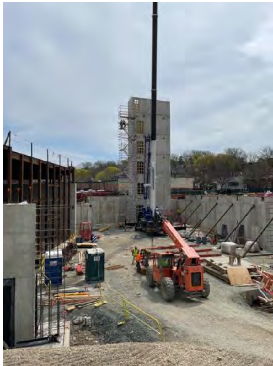
Core A forms stripped.
