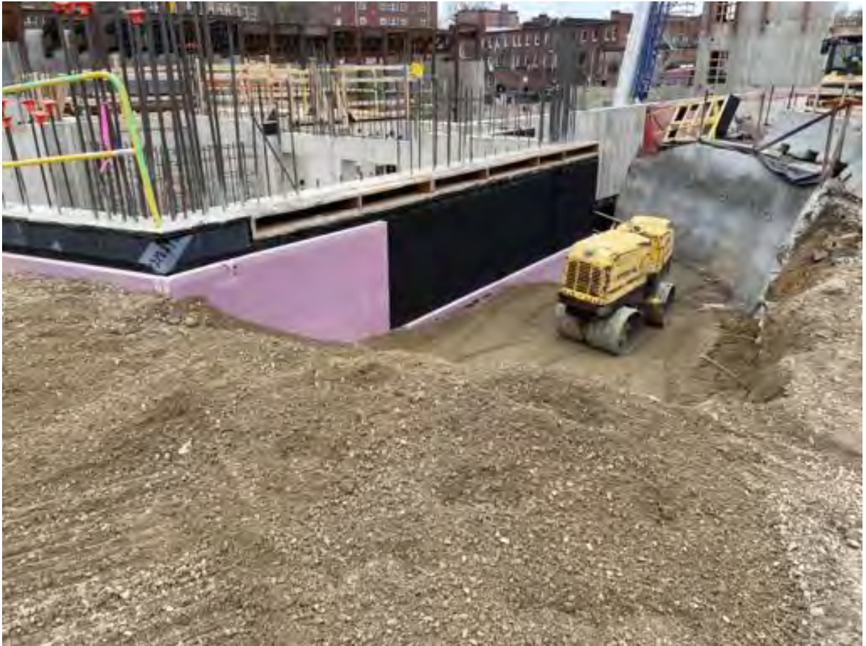
Backfill and compaction (and partial removal of SOE) at Core AB.
