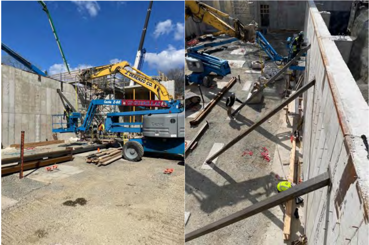
Foundation wall bracing installation.
