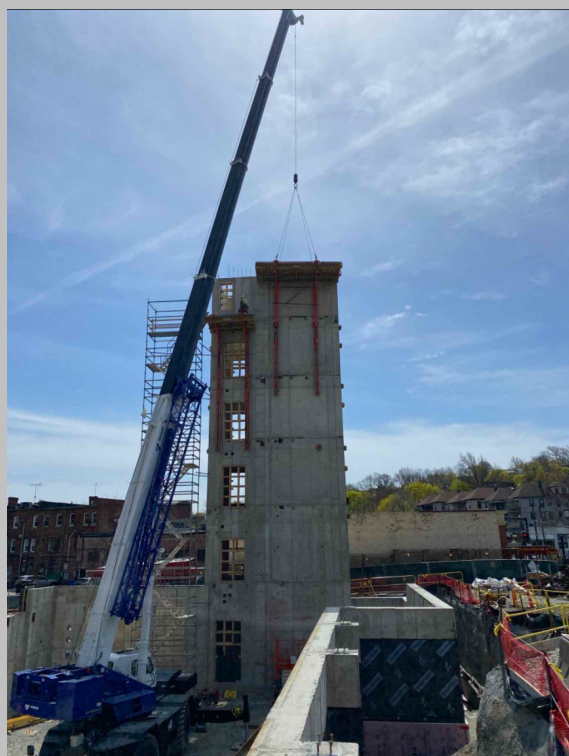
Shear Core A
