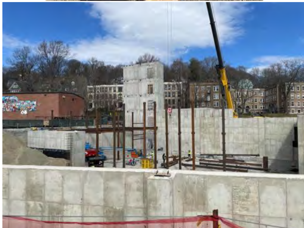
Setting steel in Area C.
