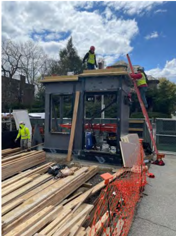
Roof work on mock-up
