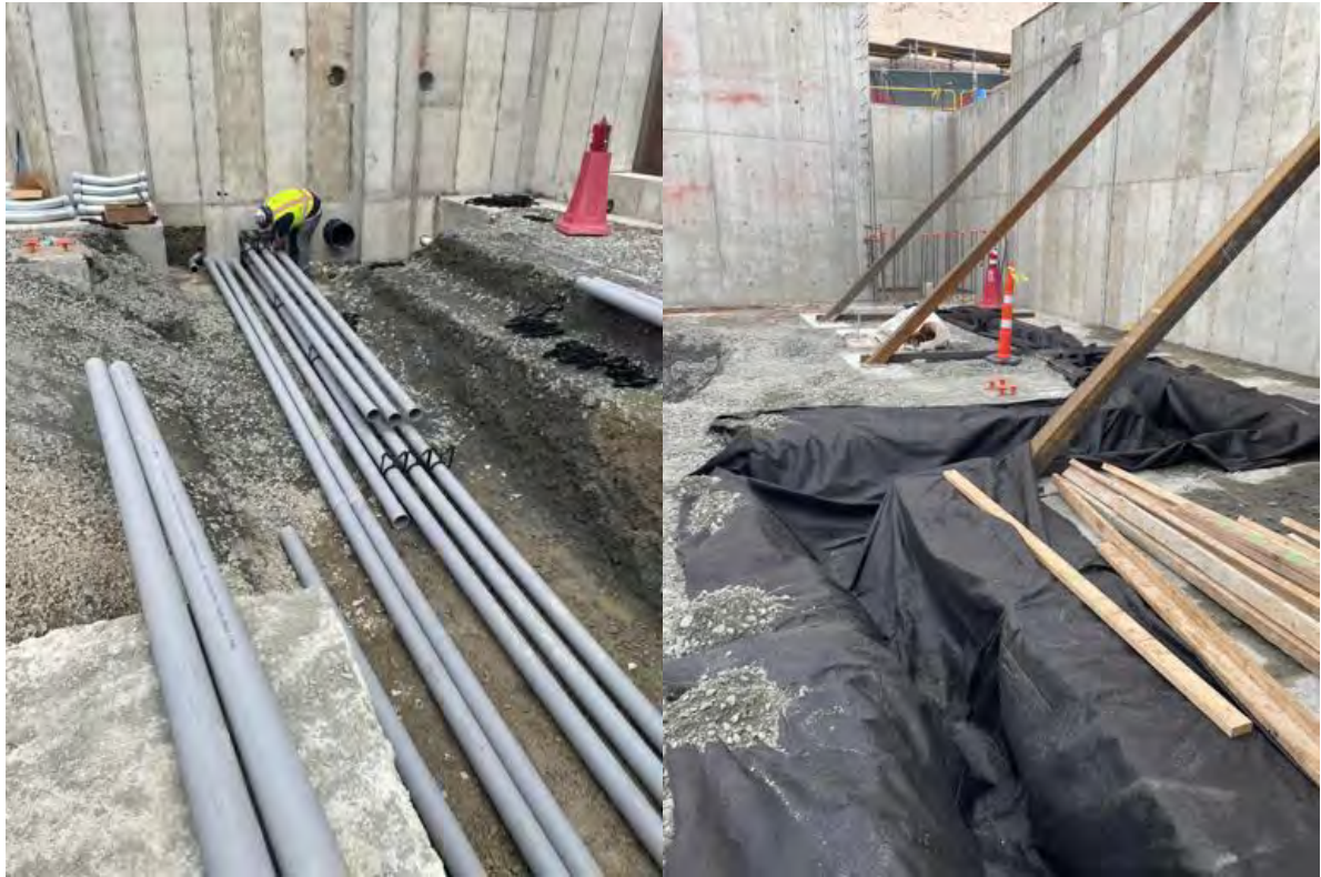
Installation of electrical ductbank and conduit.
