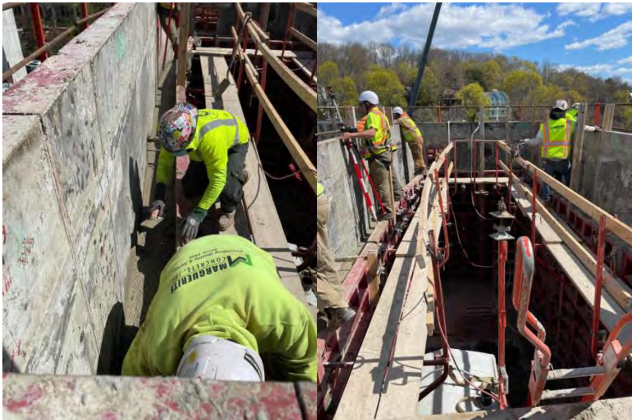
Concrete work, top of Core A.
