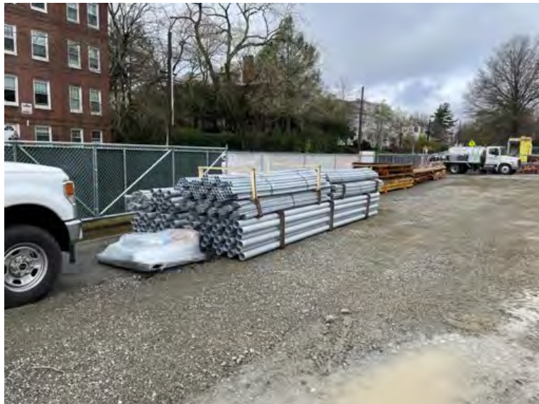
Deliveries: steel, forms, electrical pipe.
