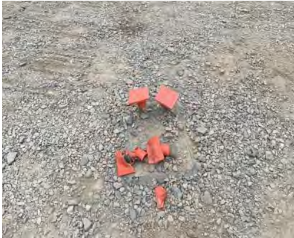
Damage to anchor bolts.
