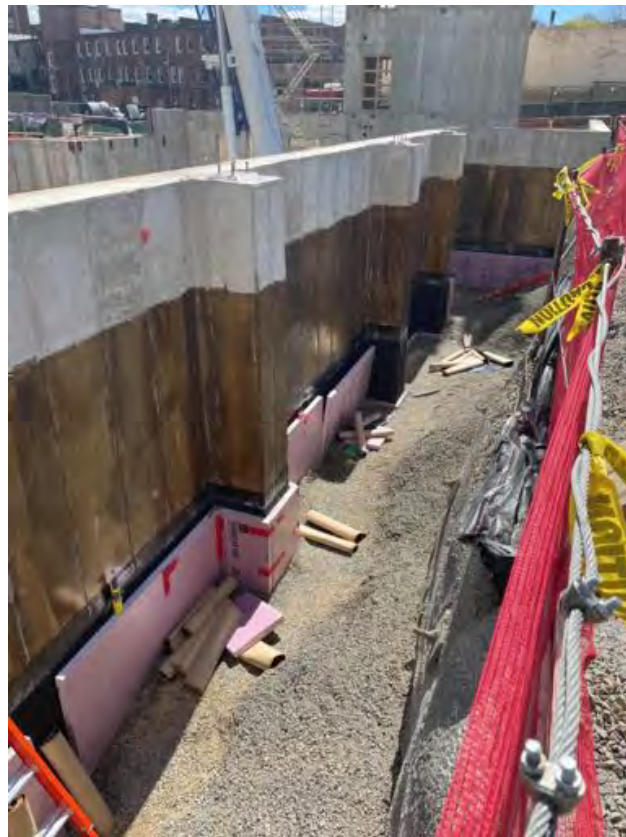
Waterproofing along line AG.
