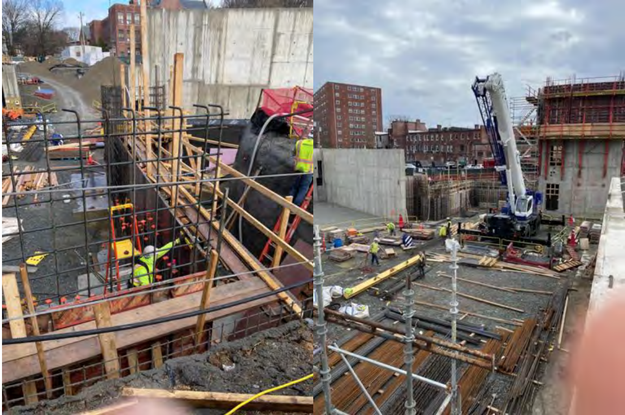
Forms ongoing at AR
