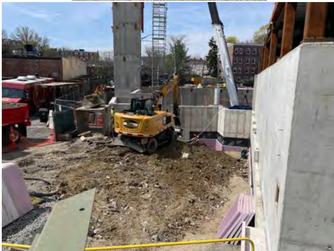
Backfill/SOE removal, East side.
