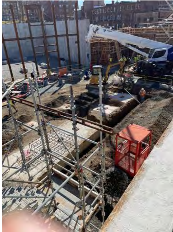
Trenching for underground utilities.
