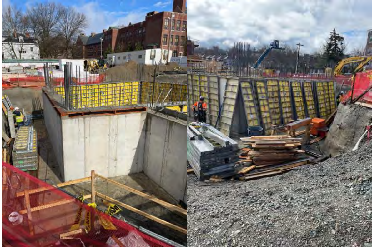
Stripped wall at Core AB
