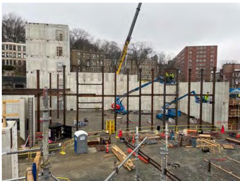
Steel installation ongoing, Sequence 102.
