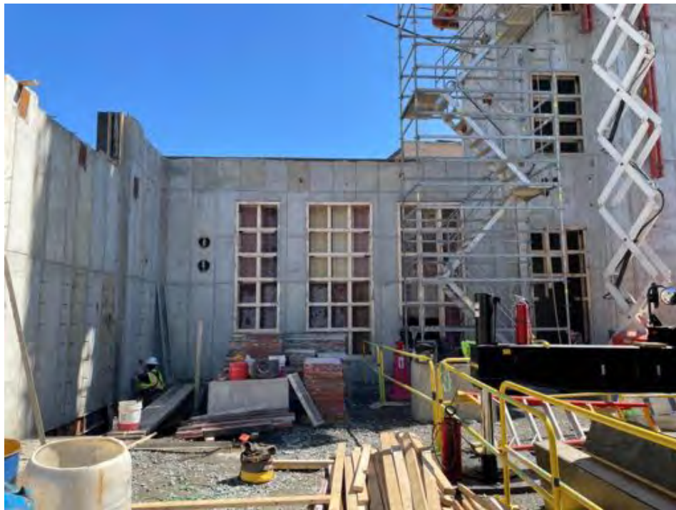
Forms stripped, line AR.
