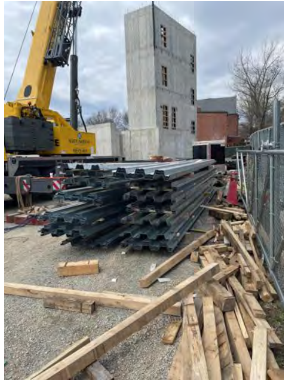
Metal deck received.
